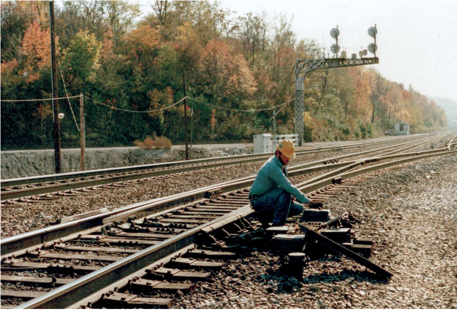
R.T. Cutcher adjusting a power switch machine, Ludlow, KY
